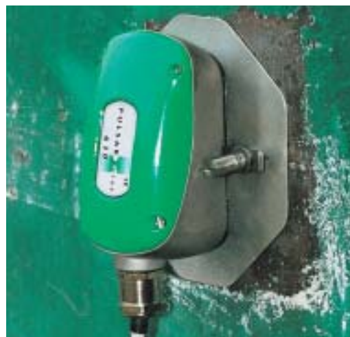
Pulsarpoint 610 attached to vessel using optional self adhesive aluminium plate
